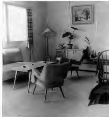
Living room. The joints between the panels are sealed with coloured plastic sections
