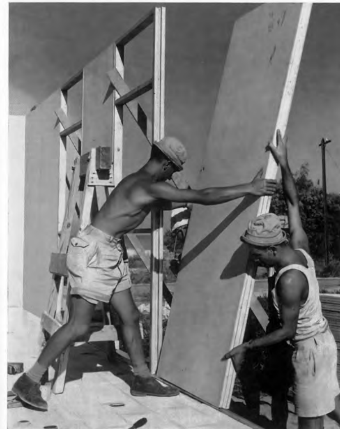
The bottom groove of the panel is inserted into the aluminium channel
